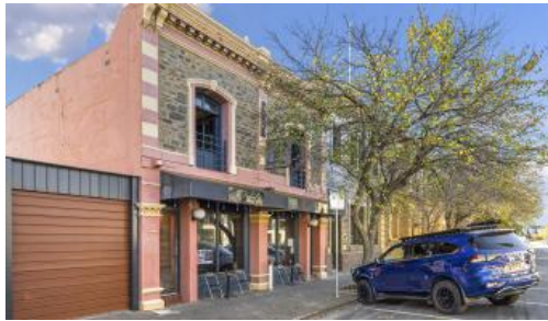
3-5 Divett Street, Port Adelaide
